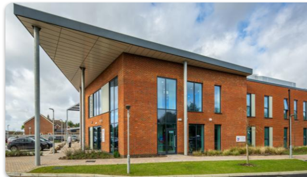
Eastergate, Croft (West Sussex) – PHP's first NZC development project
