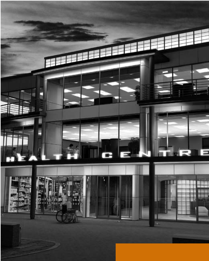
Raynes Park Medical Centre
