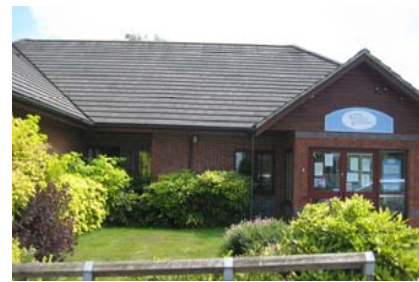
Wheathampstead Primary Care Centre
