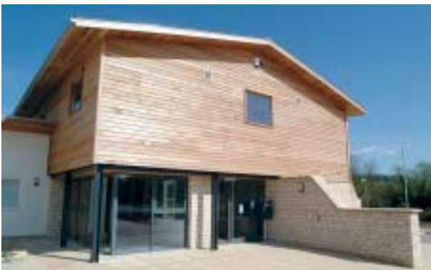
Winchcombe Medical Centre, Winchcombe, Gloucestershire Completion of New Development for a 3 GP Practice and Pharmacy
