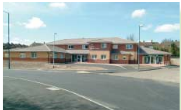
Warley Medical Centre, Oldbury, West Midlands Completion of New Development for a 7 GP Practice and Pharmacy
