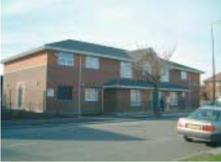
Aspley Medical Centre, Aspley, Nottingham Completion of New Development Purchase for a 4 GP Practice
