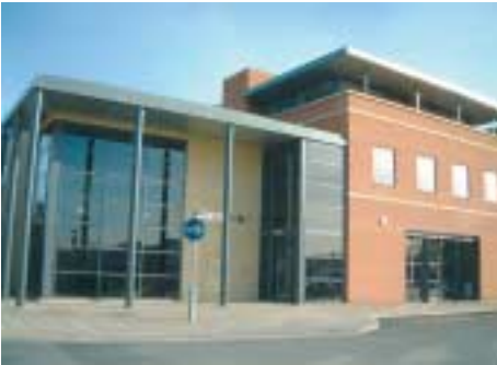
New Medical Centre, South Square, Boston, Lincolnshire Development of New Medical Practice for a 6 GP Practice, PCT and Pharmacy
