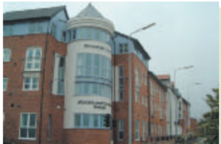
Wolverhampton Road Surgery, Stafford, Staffordshire (£1.4m) Completion of New Development for a 4 GP Practice
