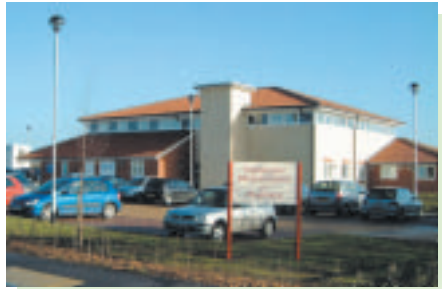
Haddenham Medical Centre, Haddenham, Buckinghamshire (£2.3m) Completion of New Development for a 4 GP Practice and Pharmacy
