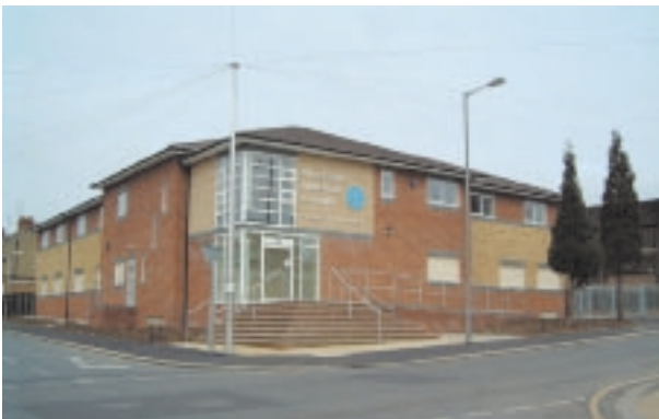
Blenheim Medical Centre, Luton, Bedfordshire (£1.9m) Completion of New Development for a 3 GP Practice
