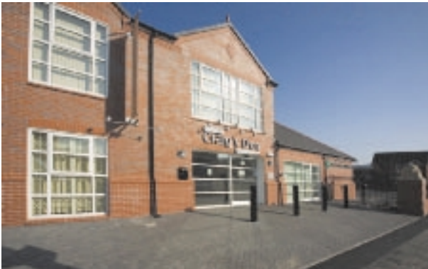
Craig y Don Medical Practice, Llandudno, NorthWales (£1.6m) Completion of New Development for a 5 GP Practice and Pharmacy
