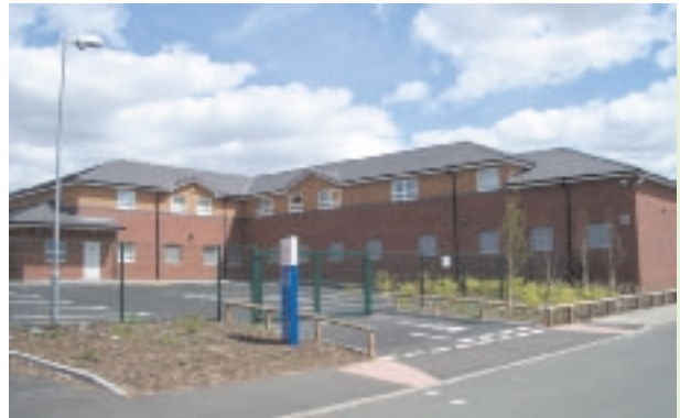
Bentley Medical Centre, Bentley, Walsall Cheshire (£3.7m) Completion of New Development for the local PCT and Pharmacy
